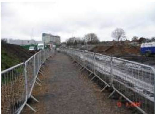
View looking west St Giles Hotel in the distance.
