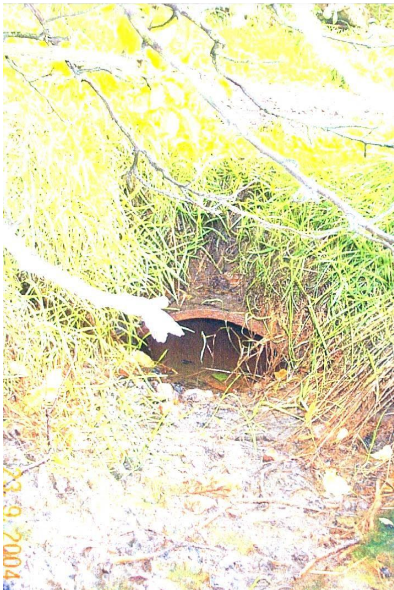
(mid field culvert of Hatton Brook)
