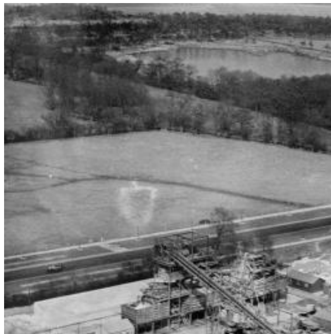
Girling Ferro Concrete Co Ltd Sand, Ballast and Gravel Works, Hatton, 1932
